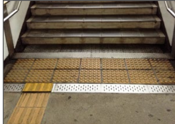
Fig. 2. TWSI before stairs, railway station Agui (Japan) Source: (Nakagoshi, 2017)
