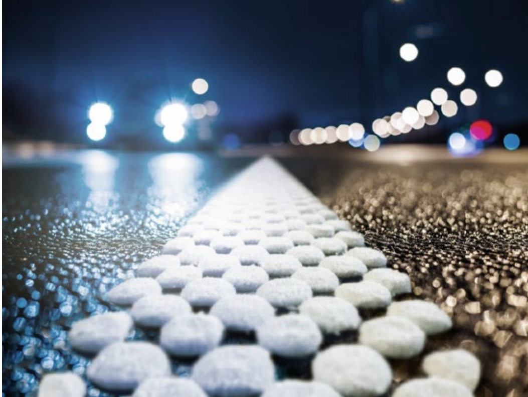
Fig. 1 Exemplary Dot-Structured Road Marking at Night Source: M. Swarovski Gesellschaft m.b.H. Used with permission.
