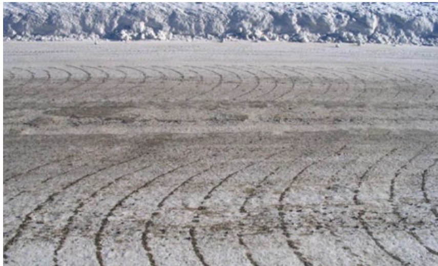
Fig. 6. The view after application of warm wetted sanding method Source: Nova Scotia Report, 2010
