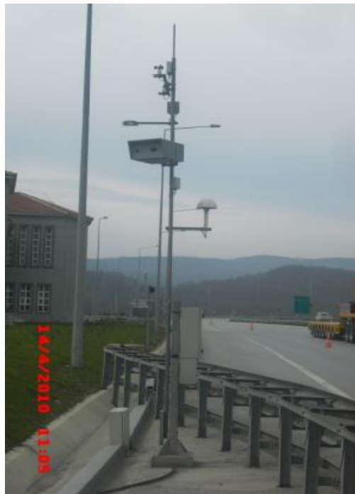
Fig. 11. Control Unit of Detecting and Preventing System at entrance of the Bolu Tunnel Source: General Directorate Highways, 2011
