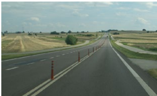
Marking with additional measures to improve road safety (high safety devices)
