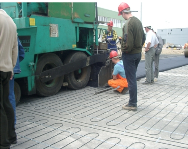
Fig. 7. Electrically Conductive Pavement implementation Source: Samm Technology Communications Industry and Trade Inc., 2014
