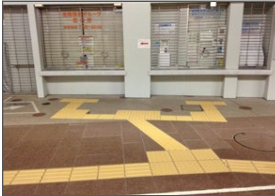
Fig. 1. TWSI in passenger hall, bus terminal Kanazawa (Japan) Source: (Nakagoshi, 2017)
