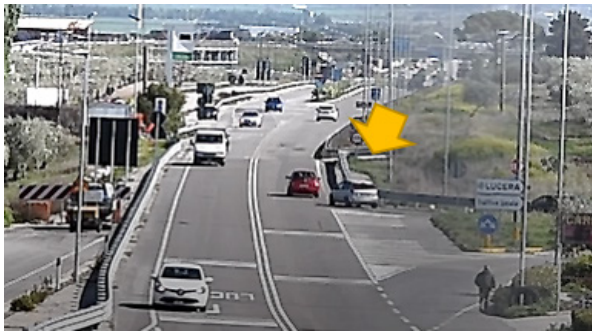
Fig. 6. Section n. 1 - Effects of the Wrong Intersection Angle
